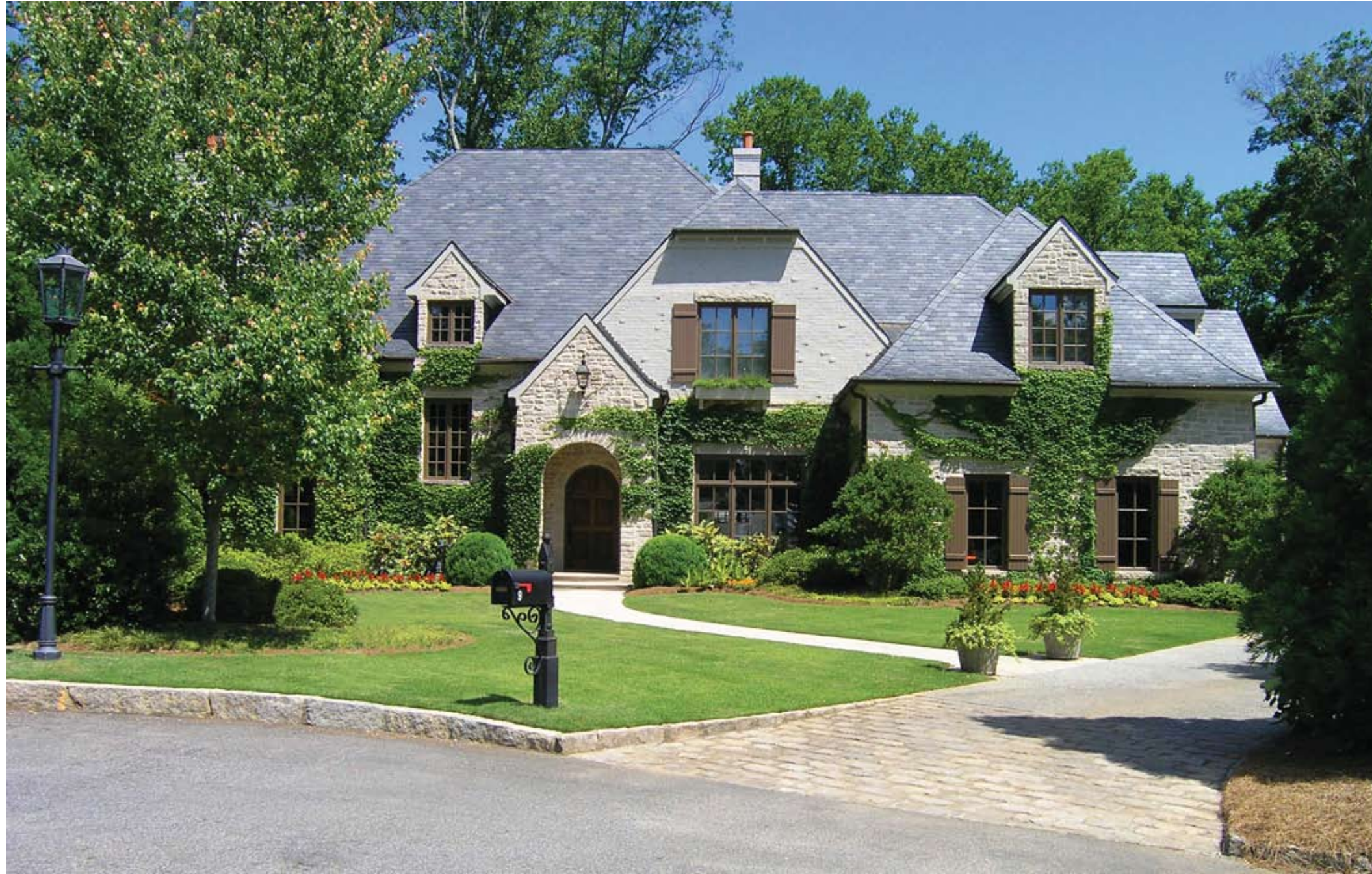
ABOVE: This romantic French Normandy country manor with its pleasing combination of tumbled limestone, painted clinkered brick and authentic Spanish slate roof is the personal home of the featured builder. Photograph by Johnson & Williams, LLC
